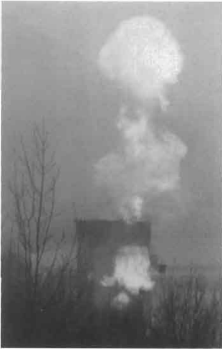
Figure 6.4 High-turbulence corn starch explosion in 500 m 3 bolted steel plate silo at Vaksdal, Norway, in April 1982 (Photographer: A. M. Fosse, Vaksdal). For a much clearer picture, see Color Plate 5.
