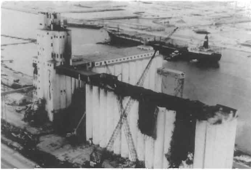
Figure 2.13 Demolished Corpus Christi grain silo plant after major grain dust explosion in 1981 (Courtesy of C. W. Kauffman, University of Michigan).
