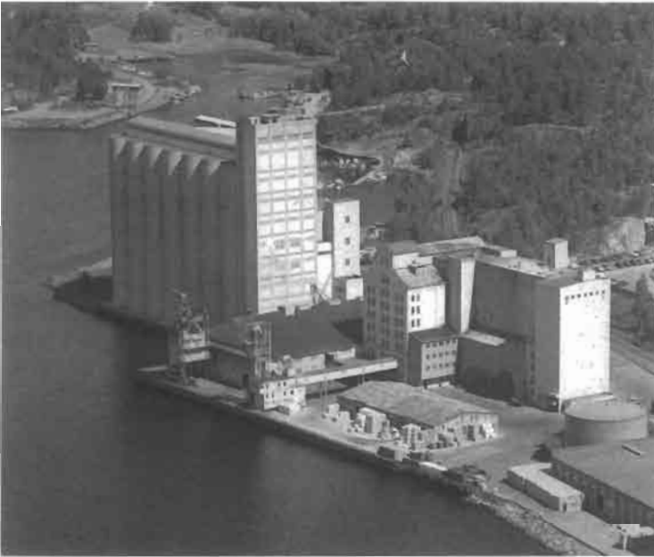
Figure 2.7 Reconstructed head house (1977) after the grain dust explosion at Kambo, Norway, in June 1976. The entire house front is covered with lightweight wall elements that can serve as explosion vent panels (Courtesy of J. Kosanovic, Kambo, Norway).
