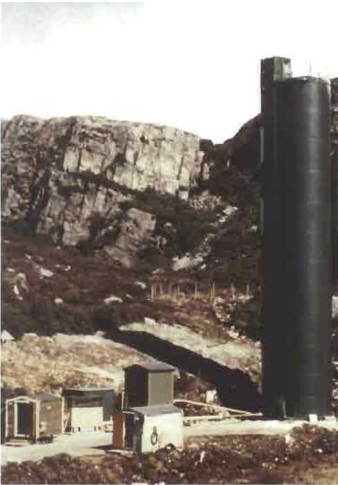
Plate 6 Experimental site outside Bergen, Norway, with 236 m 3 steel silo, dust injection system, and instrumentation cabins. Enclosed winding staircase is along the silo wall to the left.
