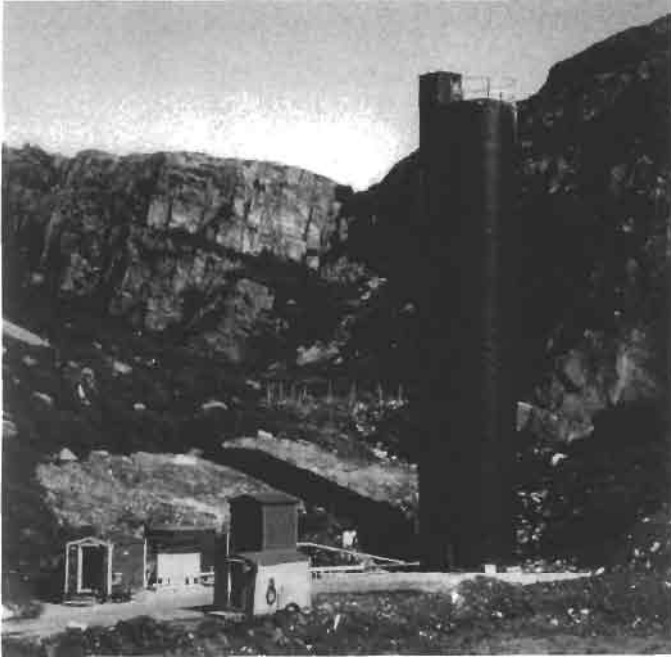
Figure 6.7 Experimental site outside Bergen, Norway, with 236 m 3 steel silo, dust injection system and instrumentation cabins. An enclosed winding staircase runs along the silo wall to the left. For a much clearer picture, see Color Plate 6.
