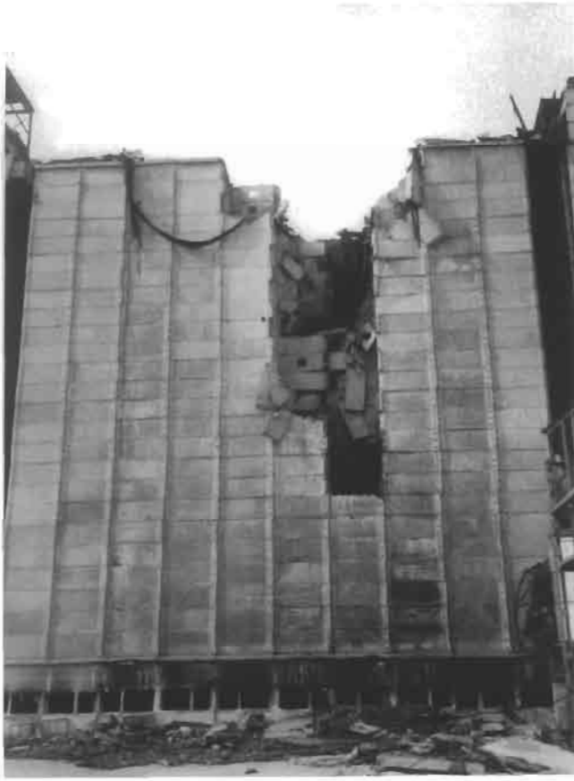
Figure 2.21 Central part of the silo complex in Tomylovo, USSR, damaged by smoldering gas explosions, 1987–1989 (Courtesy A. Borisov and B. Gelfand, USSR Academy of Science, Moscow).
