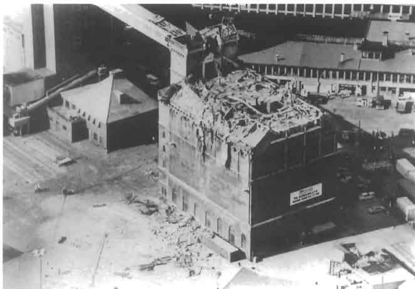
Figure 2.8 Damaged silo building after malted barley dust explosion at Oslo Port Silo in July 1976 (Courtesy of A. F. Johansen, Oslo Port Silo, Norway).
