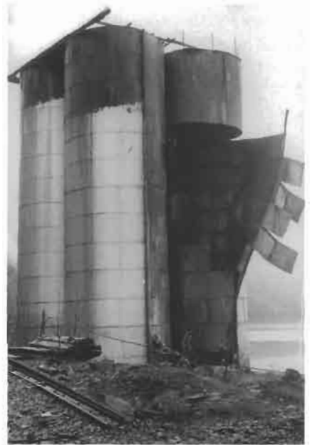
Figure 6.5 Damaged 500 m 3 silo after explosion shown in Figure 6.4.
