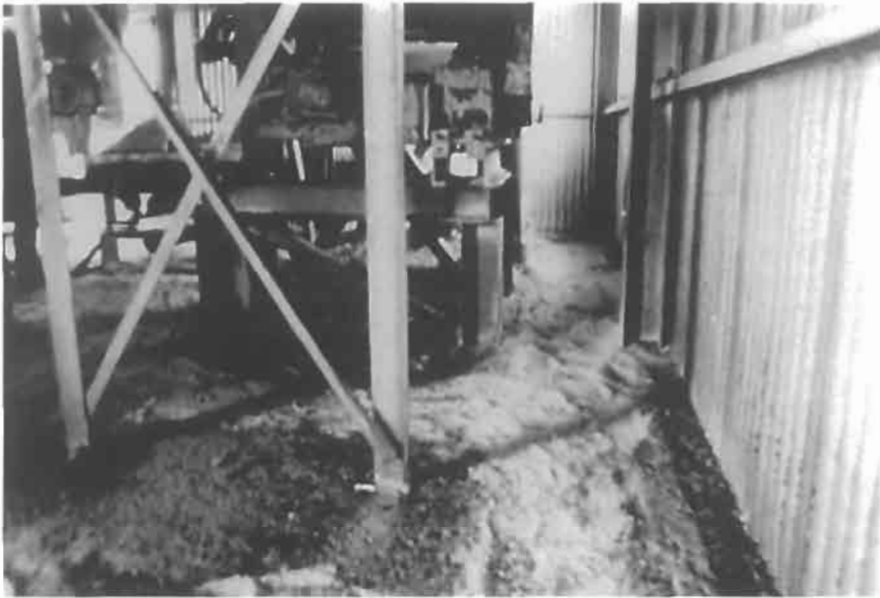
Figure 2.10 Accumulation of dust in the gallery of a river grain terminal at St. Paul, Minnesota, 1980 (Courtesy of C. W. Kauffman, University of Michigan).
