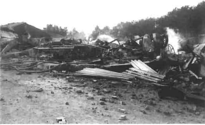
Figure 2.29 Scene of total demolition after aluminum dust explosion in the premix plant of a slurry explosive factory at Gullaug, Norway, in August 1973 (Courtesy of E. Berg, Dyno Industries, Gullaug, Norway).
