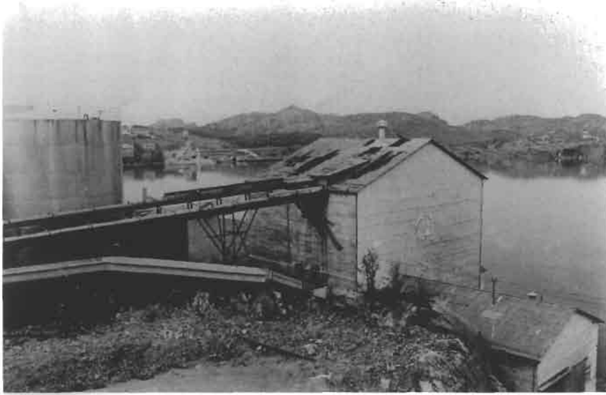
Figure 2.16 The building of the fish meal factory in Norway afflicted with a dust explosion in 1975.
